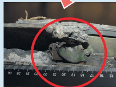
Location of the fragment in the left cockpit window frame. (Source: Dutch Safety Board)
